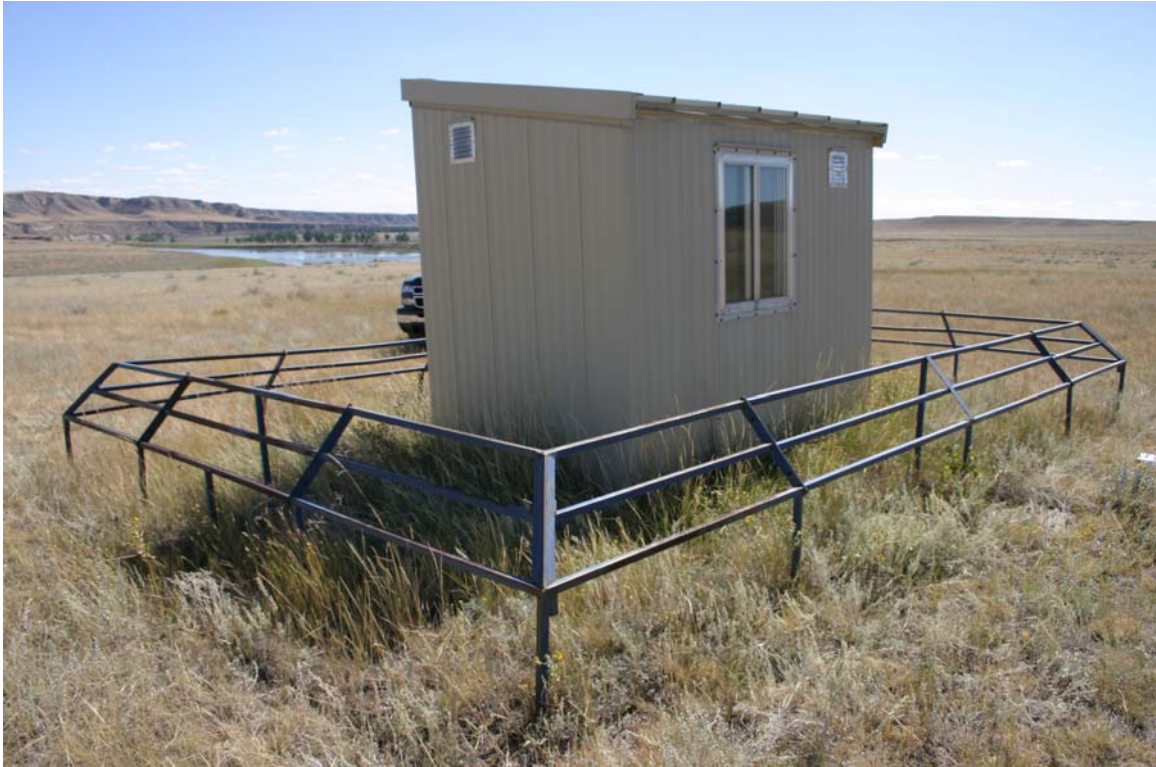
Figure 5. Photo of one type of gas development above ground infrastructure within the NWA. The shed houses the well head as well as other gas development infrastructure. The fence restricts cattle access to the shed. Cattle were frequently found rubbing similar cattle fences within the NWA, resulting in increased erosion, bare ground and invasive immediately outside of the cattle fences.
