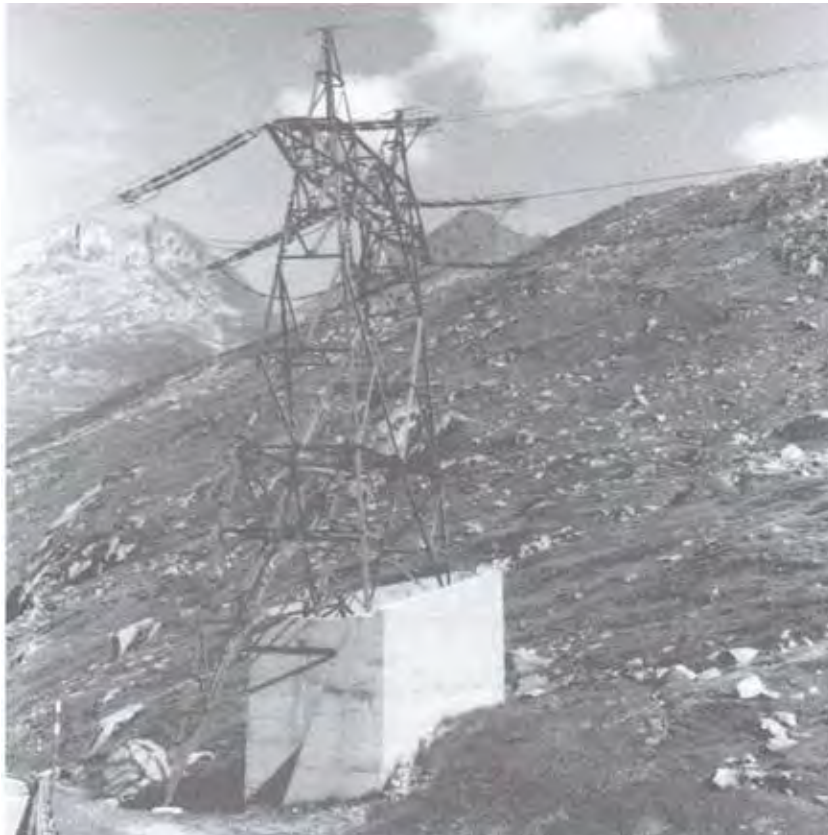
Figure 5-1. Example of splitting wedge to protect structure (McClung & Schaerer, 2006)
