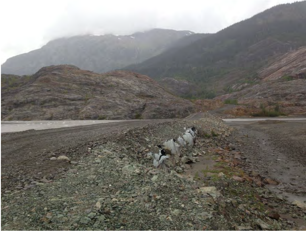
Photograph 3-1. Looking west up access road along Bowser River floodplain at approximately KP 53.7, subject to flooding and channel avulsion.
