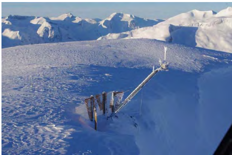
Figure 5-5. Wyssen Tower (courtesy of Wyssen Avalanche Control AG).
