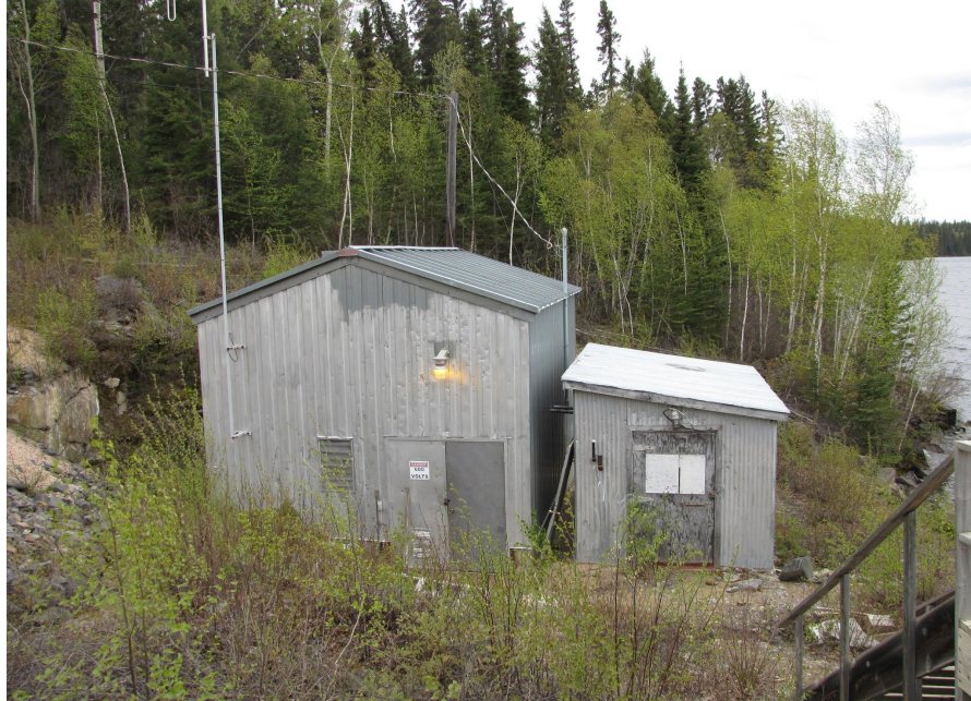
Photo 5: Snow Lake Pumphouse
