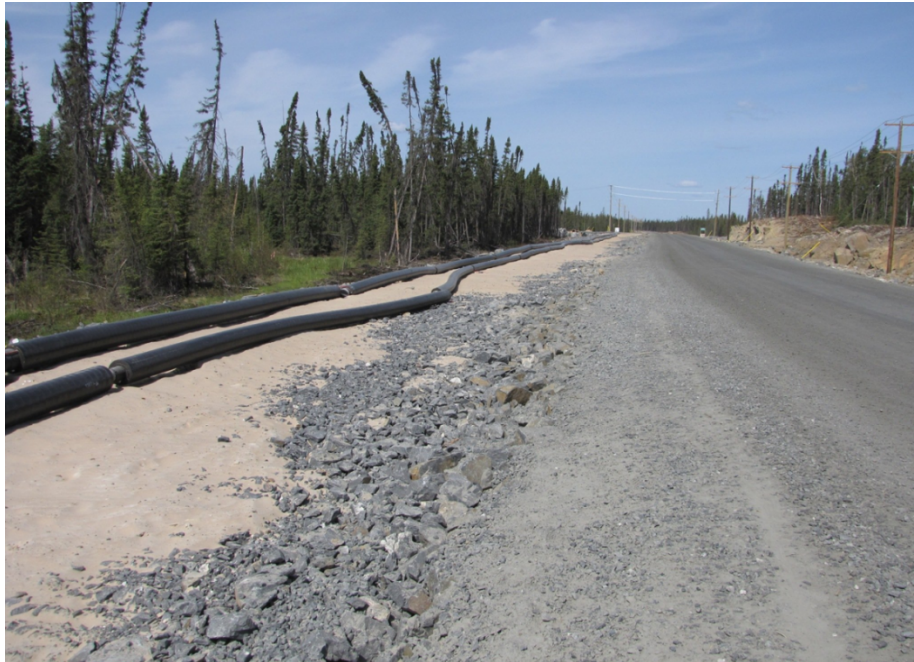
Photo 3 - Corridor of the Pipeline System (along the Lalor Access Road from Lalor site to PR 395).
