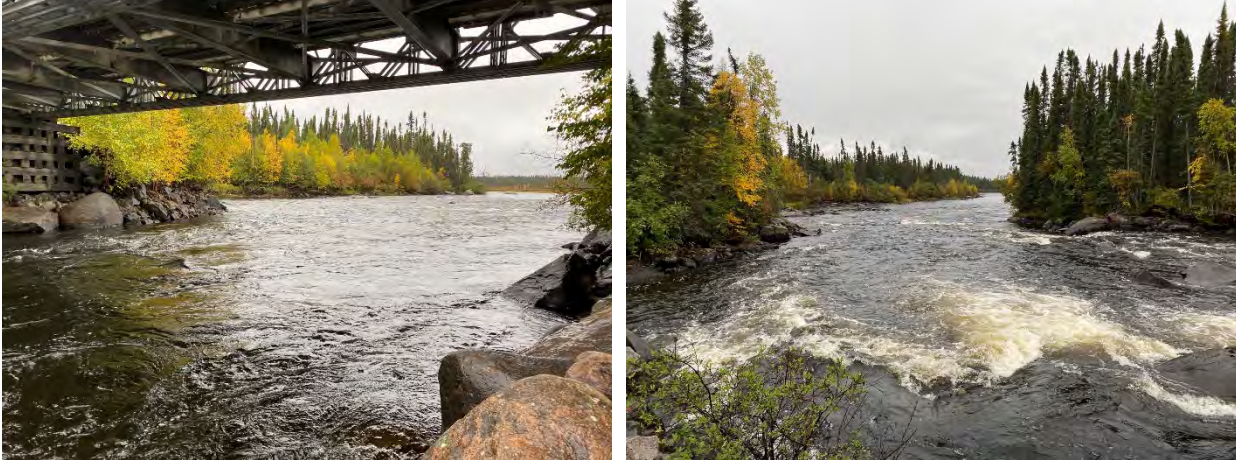
Figure 2 Proposed discharge location is located immediately upstream of the Hughes River bridge. Photo on the left is looking upstream from the north abutment of the Hughes River bridge, near the proposed discharge location. Photo on the right is looking downstream from the north abutment of the bridge, immediately downstream of the proposed discharge location.
