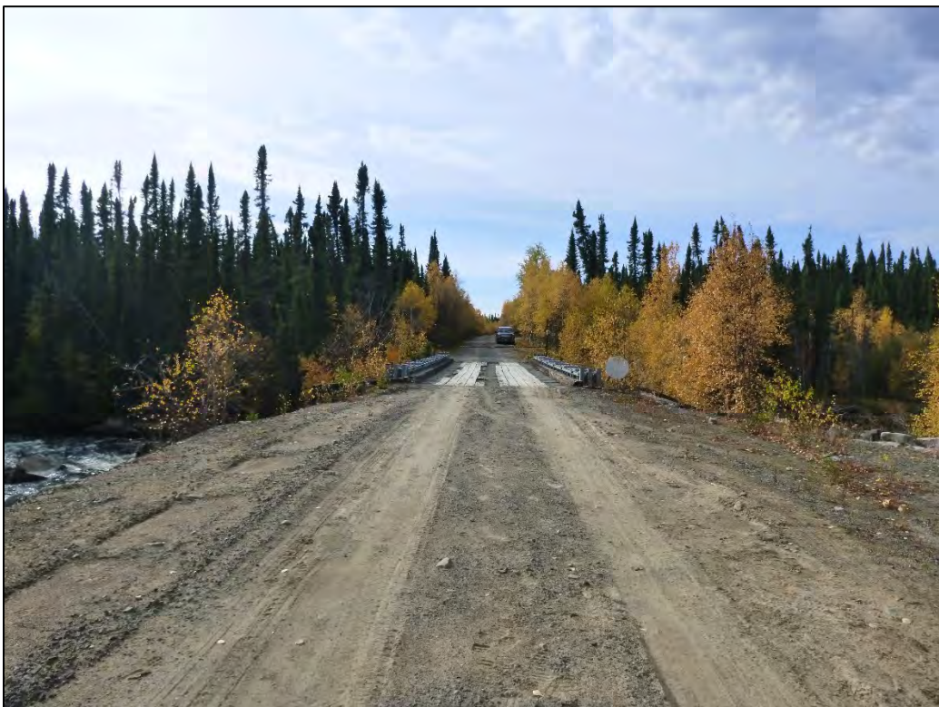
Photo 2: Hughes River Bridge crossing
