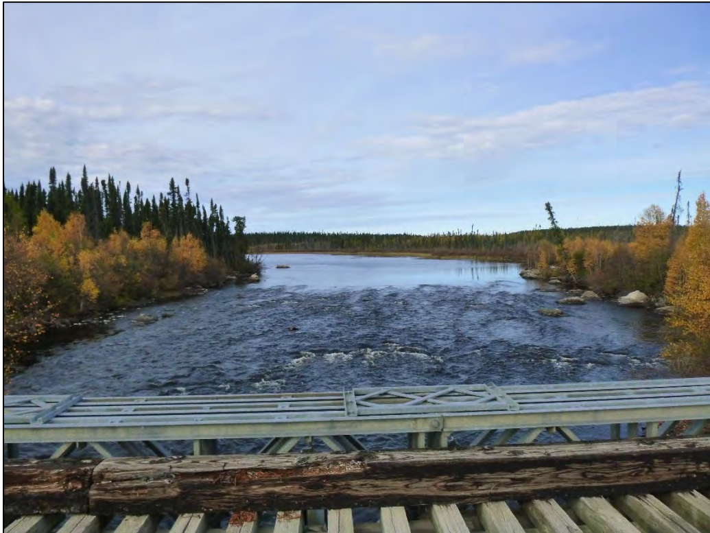
Photo 4: Hughes River Bridge crossing – looking upstream
