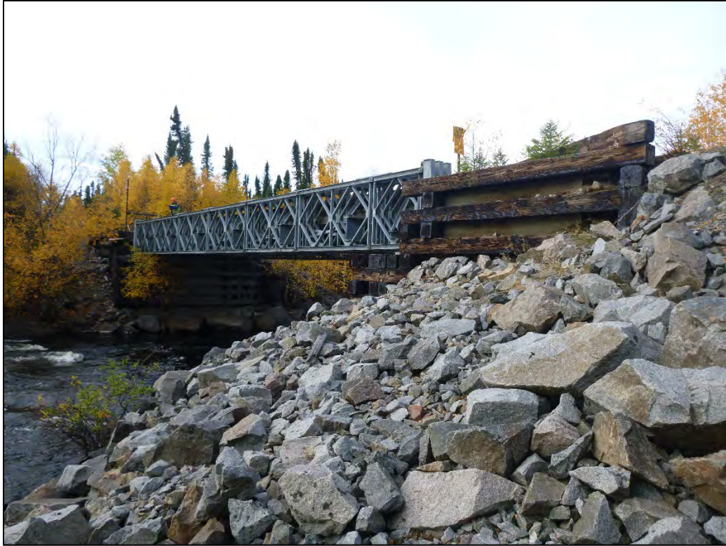
Photo 3: Hughes River Bridge crossing – side view
