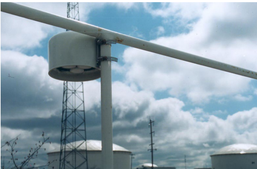
Figure 2: Rain Shelter In Place
