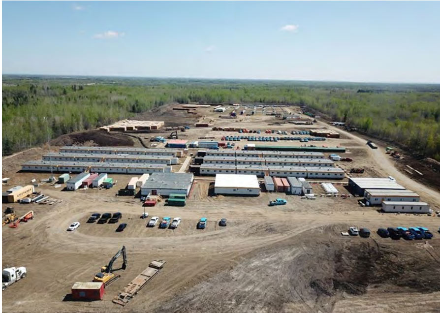
Figure 6-6: Typical Layout of Temporary Construction Camp and Laydown/Storage Area (AtkinsRéalis, 2024g)
