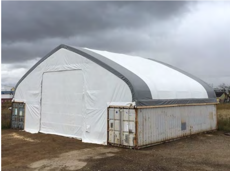
Figure 2. Enclosed Industrial Tent
